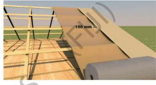
4. Allow 150 mm overlap at joins (50 mm is adequate when joins are to be taped).
