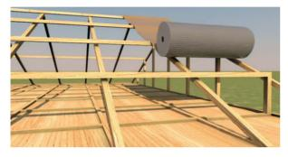
1. Roll out the Kingspan AIR-CELL <sup>\*</sup> product from the ridge to gutter, over and perpendicular to the roof battens.
