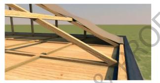
2. Ensure a 50 mm overlap into the gutter and a nominal 40 mm sag between battens is achieved.
