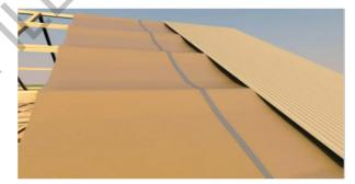
5. End joins should be overlapped by 600 mm if not taped.
